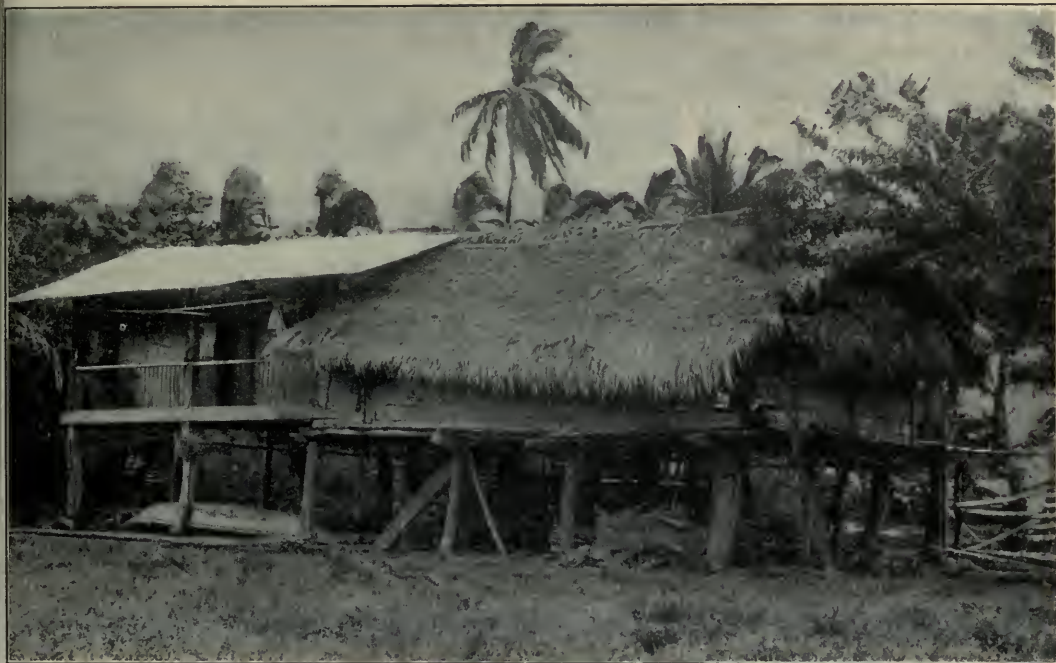
FIG. 442.— A house in Ecuador raised above the ground because of the dampness.
